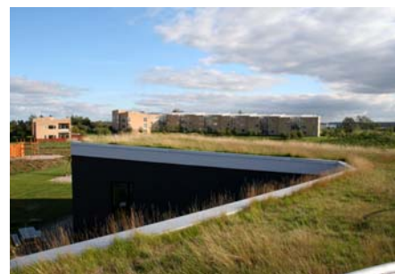
The roof of the day-care centre has an inclination of roughly 3%.
