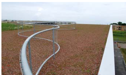
The roof is accessible up to the curving fence.
